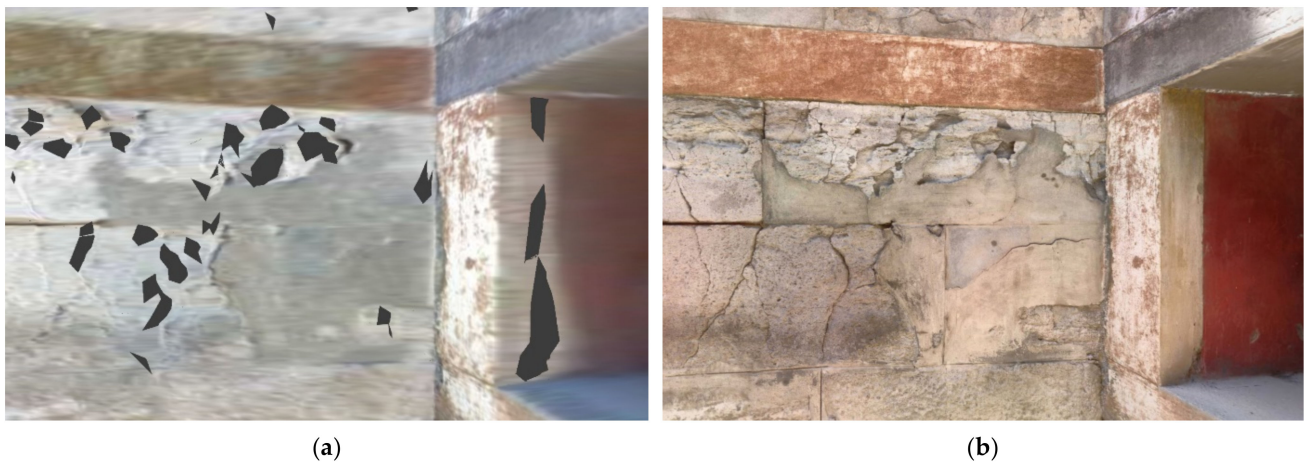
Figure 15. Preserving accurate texture information by maintaining the quality of the most perpendicular and close-proximity scans on top of an average image-stacked texture: (a) panoramic projection with an example with an acute angle 6 m away, and (b) panoramic projection with an example with a distance of 1.5 m, which was mostly perpendicular.
